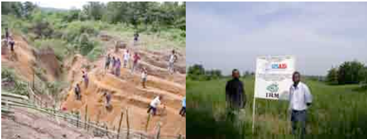
Slope preparation on the left, and the final product after 4 months on the right with the Alain Ndona (right of the sign) who worked with the community on this gully reclamation.
